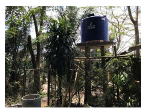
Roughly a week ago, our contractors completed the construction of our water tower. It stands at just over 3 meters tall and can hold 2,000 litres.
