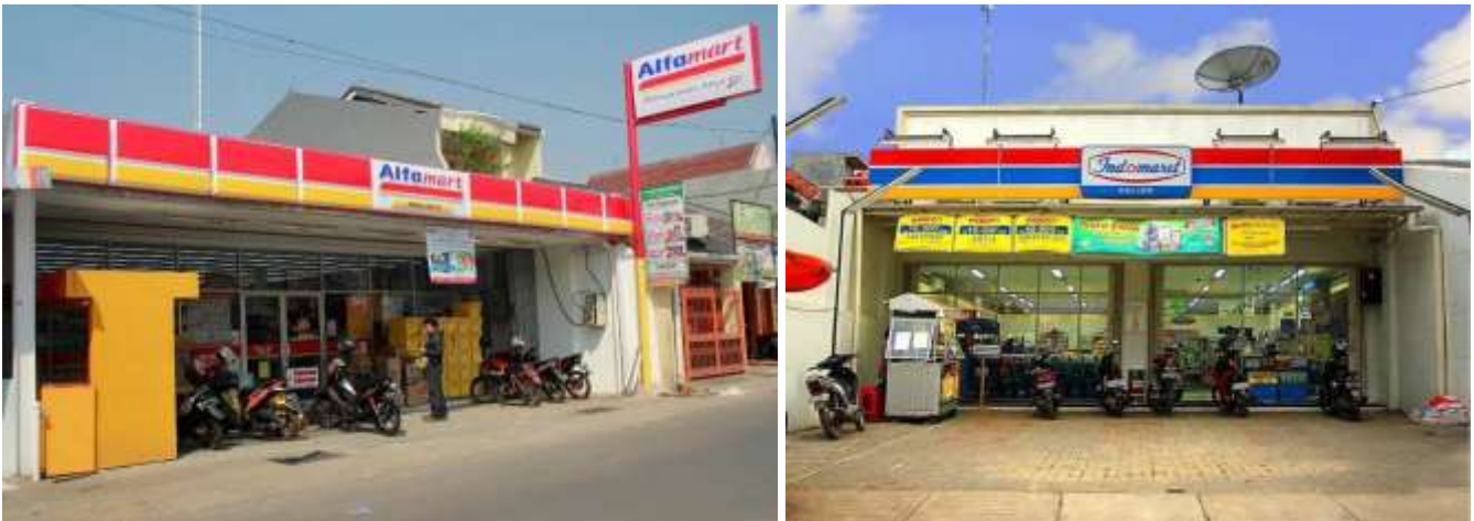
Typical shop fronts
